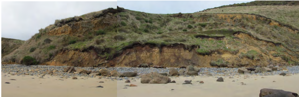
Figure 5. The large slip in the middle of the bay.
