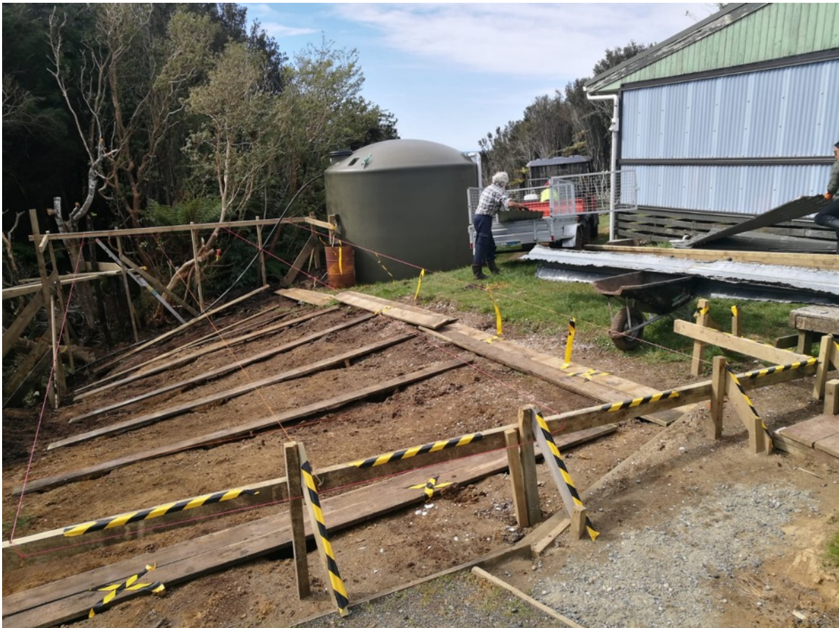
Foundation preparations for the new bunkhouse
