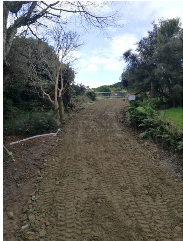
Upgraded vehicle access track
