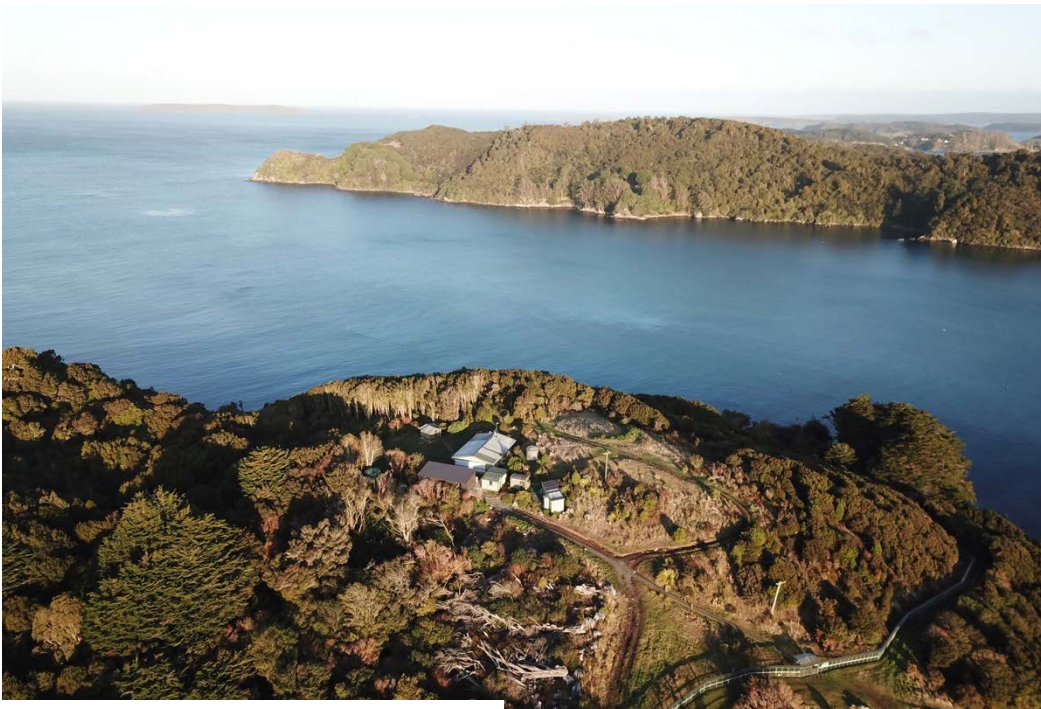
Mamaku Point school camp facility
